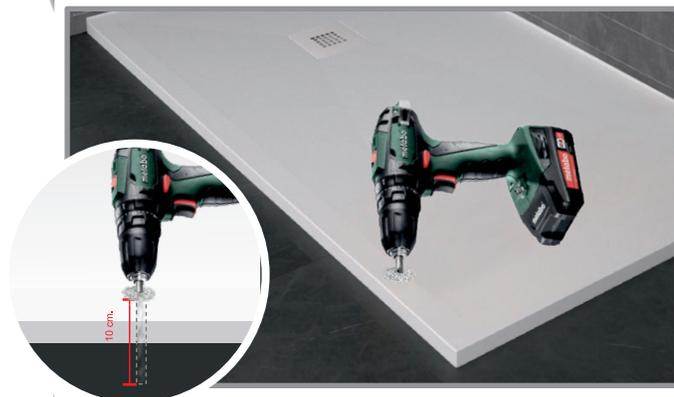
**3** Replace the drill bit with one suitable for the floor material on which it has been installed and continue drilling the floor underneath to a total depth of 10 cm.
