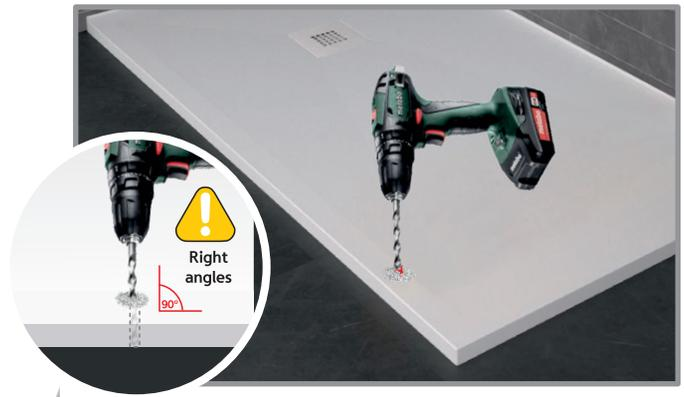
**2** Drill with a **hammerless drill** using the 8 mm drill bit supplied. The drill bit must drill through the entire shower base. **Drill always at right angles.**
