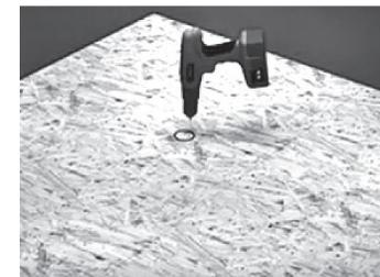
En: Once location for drain is identified, cut a 3-1/4" to 3.75" hole in the substrate, and install drain body support with modified thin set mortar.
